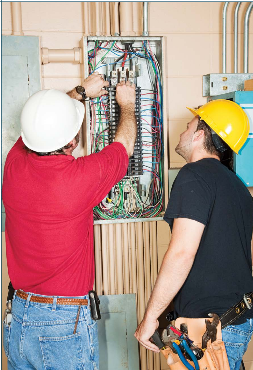
The electrician in the yellow hat is learning about circuit breakers.
